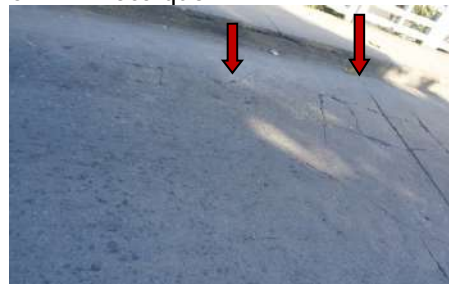
Figura 24 – Recalque
